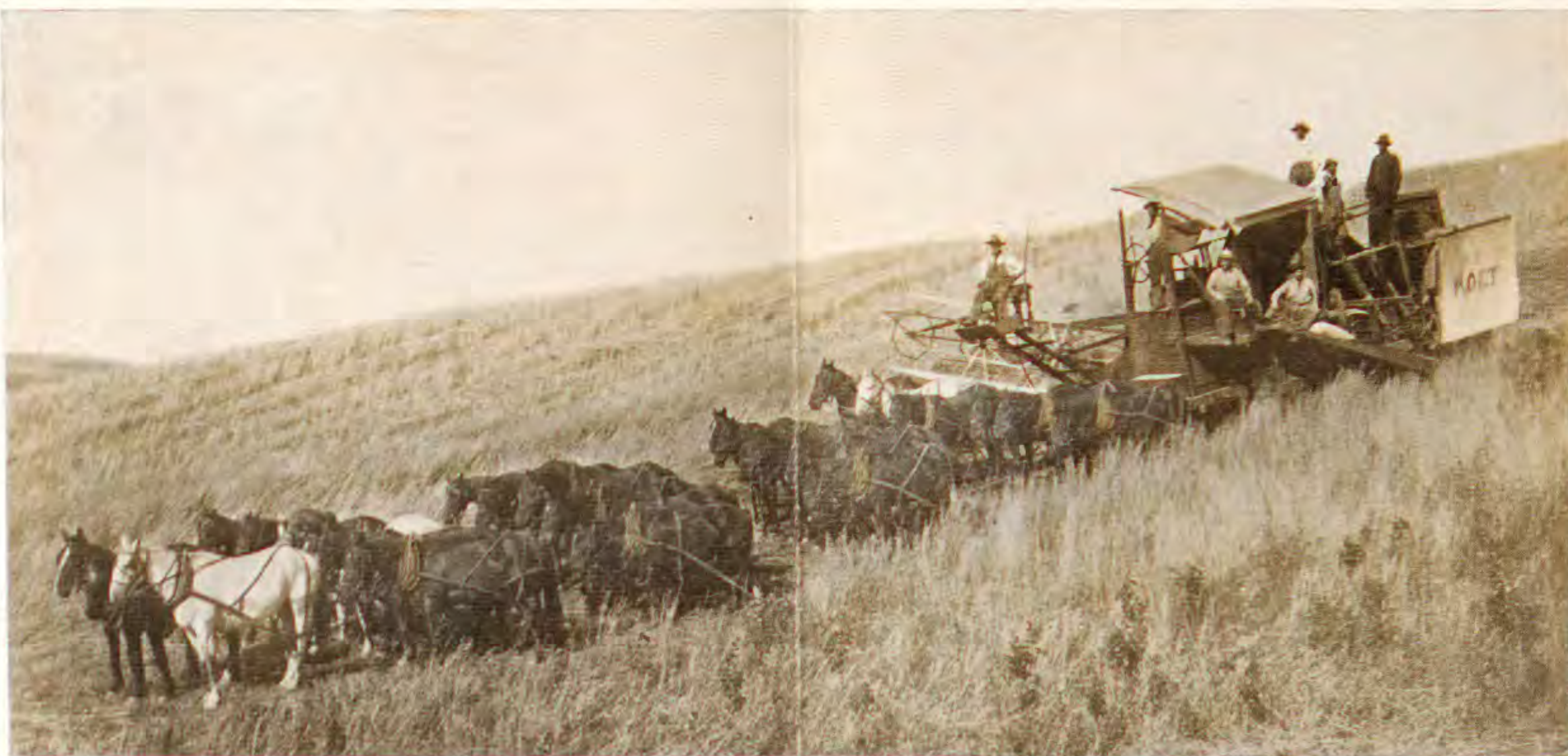
Nearer view of the great "Combine." In one operation it cuts a swath from 12 to 18 feet wide and delivers the grain in sacks.
