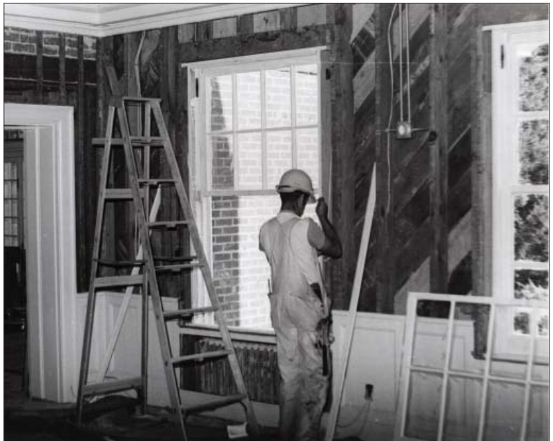
Renovation finally gets under way in the Mansion. Washington State Archives
