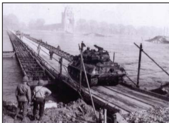
Crossing the Rhine River in Germany on a pontoon bridge, April 1, 1945. The haze is caused by smoke generated by U.S. Engineers to prevent enemy aircraft from locating the bridge.
